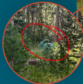
Propane tank without 10' clearance
